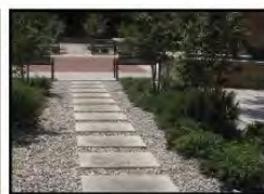
CONCRETE PAVERS IN GRAVEL
